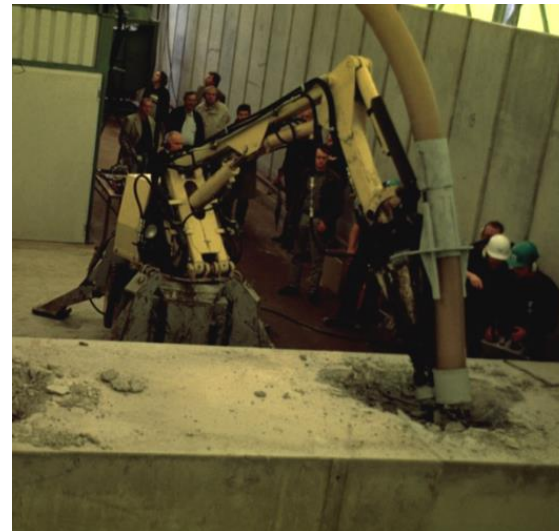
Decommissioning of heavy concrete ceiling for research reactor KNK
