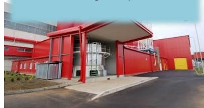
Facility for Final Treatment and Conditioning of Liquid RAW
