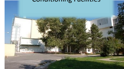
RAW Treatment and Conditioning Facilities
